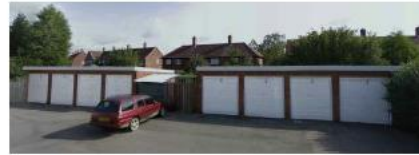
EXISTING SITE PHOTO
